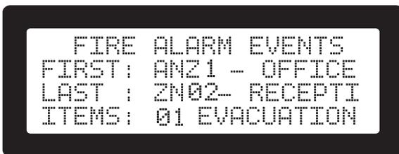
Figure 32. Default alarm indication with evacuation screen
